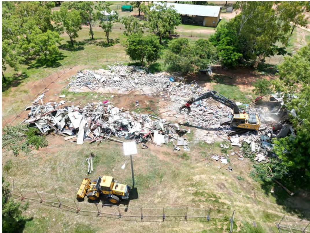
Jawoyn Contracting Works in Wugularr (Beswick)
