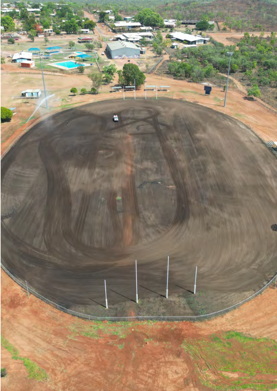
Ngukurr Oval Project – Oval Resurfacing
